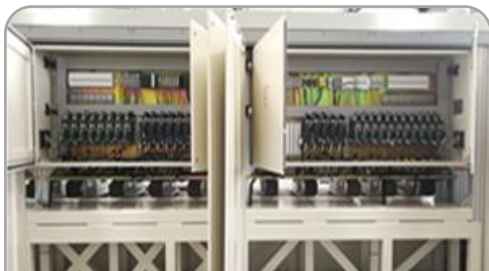
Isolated Electrical Cabinet
